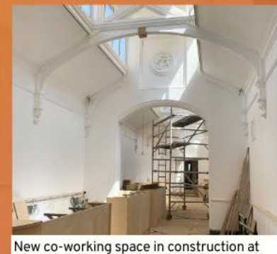
New co-working space in construction at Stanley Arts
