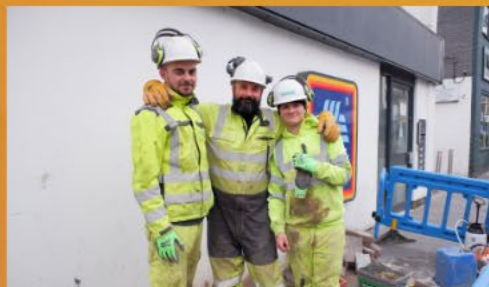
Installing a new market power supply on Station Road
