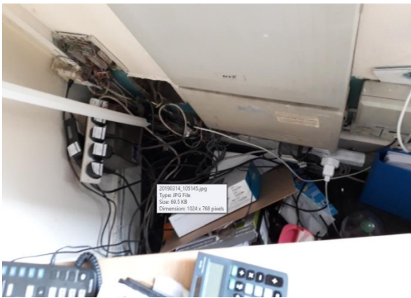
< Condense dropping on outlets not IP rated.
