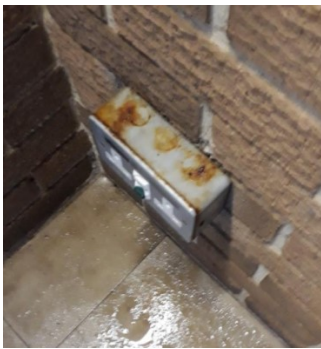
< Condense dropping on outlets not IP rated.
