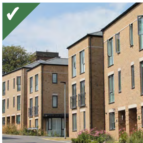
Figure 2.27b: Example of where placement of servicing items has been considered early in the design development, ensuring elevations are free of clutter.
