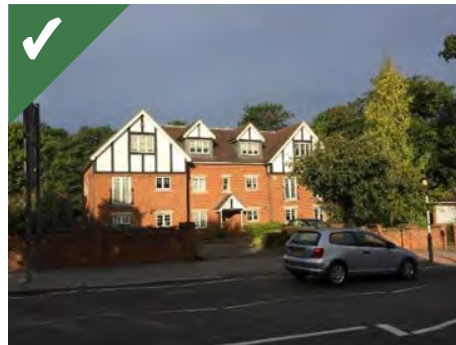
Figure 2.17c: A wide development which has successfully dealt with its width through proportions and fenestration.
