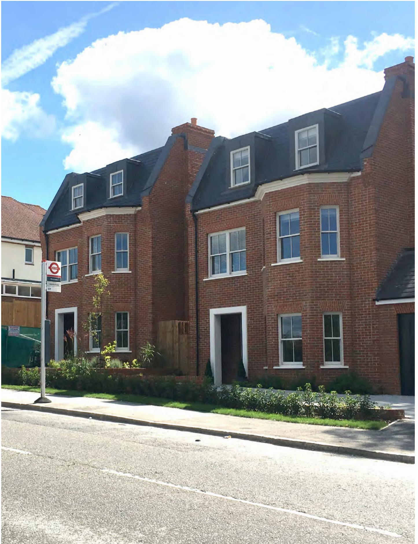
Figure 2.19a: A street facing development of family homes on Purley Downs Road. The development provides accommodation within a mansard roof.
