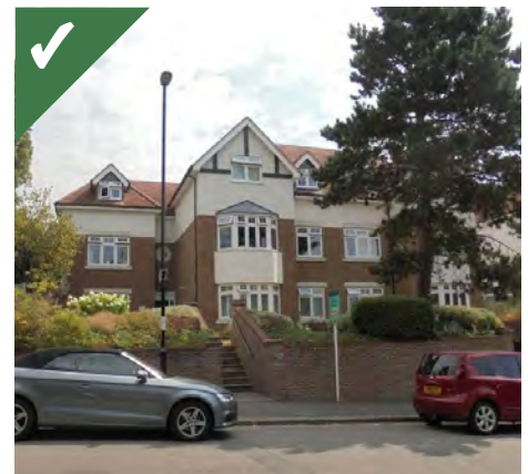
Figure 2.29d: The impact of a retaining wall is minimised through the use of planting.
