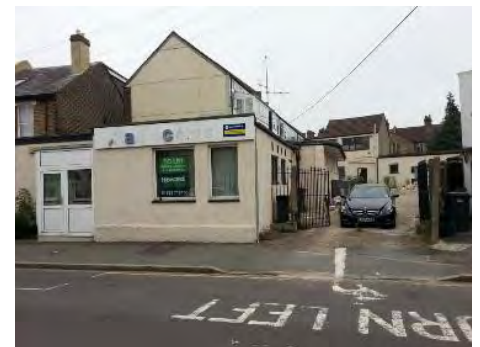
Figure 2.5a: Oval Mews, before redevelopment with a change of use.
