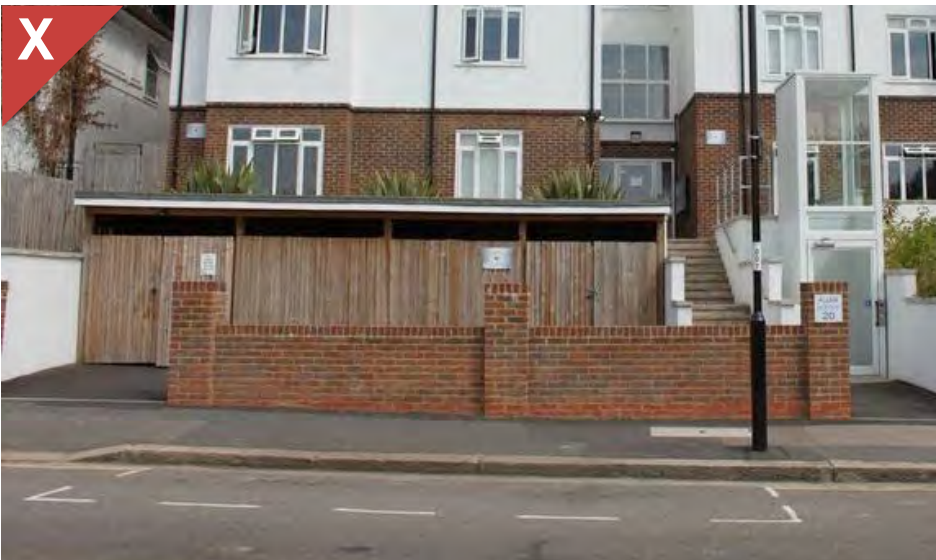
Figure 2.31c: Refuse stores in highly visible locations that are not integrated into the landscape design or any other aspect of the design.
