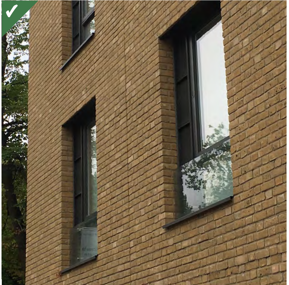
Figure 2.25a: Deep reveals provide a sense of solidness that can add appeal to facades.
