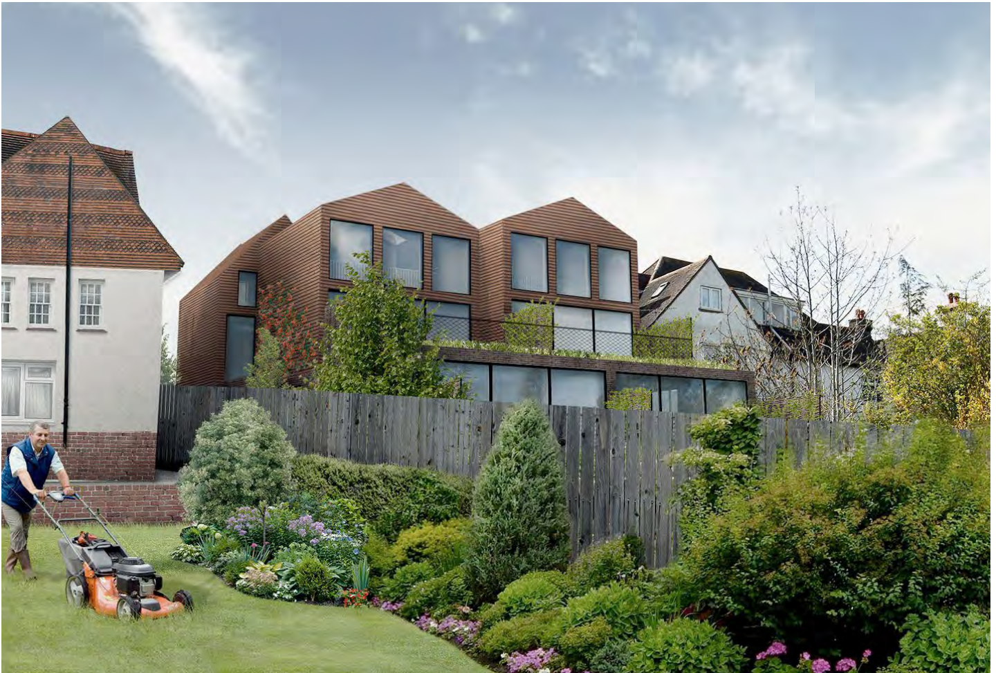
Figure 2.11a: A proposal designed by MATA Architects that steps in from the boundary and down in height where it extends beyond the rear of the neighbouring properties.
