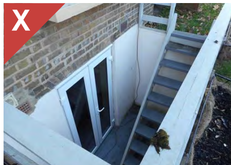
Figure 2.20d: Poorly designed and small lightwell that is not integrated into the design of the wider proposal.
