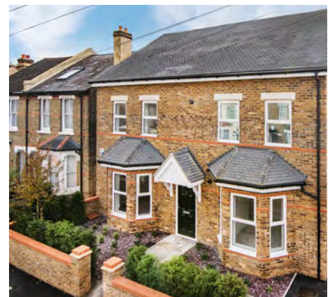
Figure 2.22c: Faithful replication of material and detailing in a street facing development. (Photo: Chartwell Land & New Homes)
