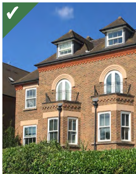
Figure 2.26b: Balconies facing the street that are successfully integrated into the design of the proposal.
