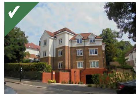
Figure 2.20e: Successful use of topography to integrate parking into a basement. Once matured, planting will reduce appearance of retaining wall.
