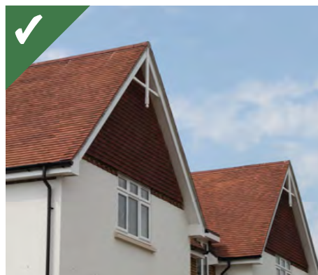
Figure 2.19e: Pitch of roof is steep enough to read positively in the streetscene.
